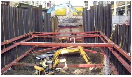
The contract was undertaken to allow a 200 tonne body panel Press to be installed in the car assembly plant to provide additional press capacity. During the tender period we reviewed various excavation support and recycling tunnel construction solutions to identify the most cost effective and least disruptive techniques.
